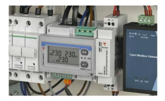
Just a single click is required to connect the multiple current transformer blocks to the meters, zeroing connection errors. The CT ratio is automatically read and set.
